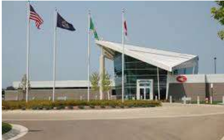
MA 52 TERMINAL- AIRPORT
