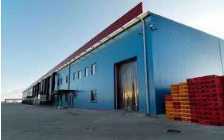
MA 74 COLD STORAGE
