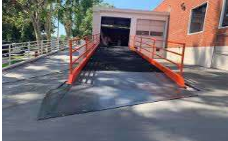
MS 132 LOADING RAMP
