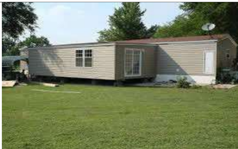
MS 41 MOBILE HOME ADDITION
